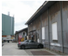
Before Photograph - Reference F3916 2014
