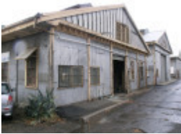
FORMER MELBOURNE HARBOUR TRUST WILLIAMSTOWN WORKSHOPS SOHE 2008
