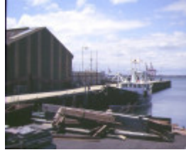
1 former melbourne harbor trust workshops ann street williamstown boyd jetty jan1999
