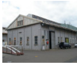
Before Photograph - Reference F3916 2014
