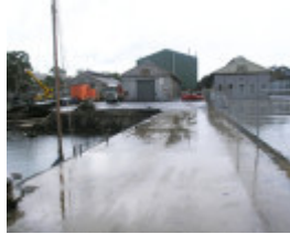
FORMER MELBOURNE HARBOUR TRUST WILLIAMSTOWN WORKSHOPS SOHE 2008
