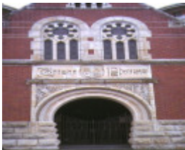
bairnsdale courthouse nicholson street bairnsdale entrance detail
