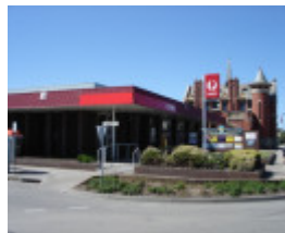
Bairnsdale courthouse nicholson street bairnsdale behind modern PO replacing AJ Macdonald-designed post office
