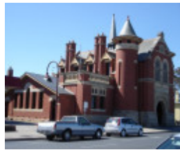
H1462 Bairnsdale Court House from the SW
