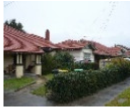
Somali Street south side
