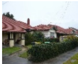
Somali Street south side
