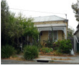
Dudley Street Precinct - 9 Dudley Street
