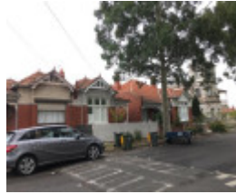
Dudley Street Precinct - 47- 51 King Street
