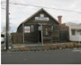
Church (former), 170 Albert St Brunswick
