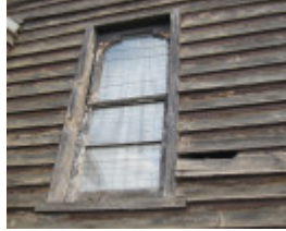
Church (former), 170 Albert St Brunswick
