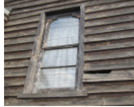
Church (former), 170 Albert St Brunswick
