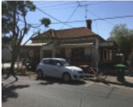
Shop - 103 Albion Street
