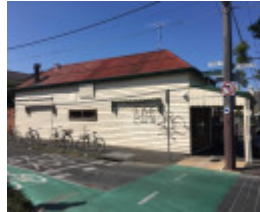
Shop - 103 Albion Street
