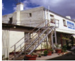
guildford hotel music hall & stables midland hwy guildford rear view of hotel
