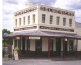
1 guildford hotel music hall & stables midland hwy guildford front view of hotel
