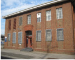
Telephone Exchange - 3-5 Frith Street, Brunswick
