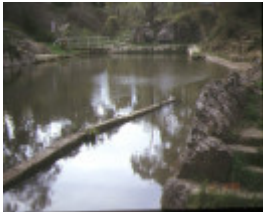
hepburn swimming pool interior wall ms sept1999
