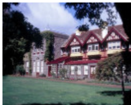
h00289 1 murndal murndal road hamilton homestead
