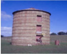
h00289 murndal murndal road hamilton silo
