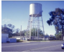
h01833 water tower and tank millard street wangaratta view from street she project 2003
