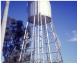
h01833 water tower and tank millard street wangaratta tower and pipeworks she project 2003
