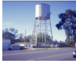
h01833 water tower and tank millard street wangaratta view from street she project 2003
