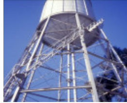
h01833 water tower and tank millard street wangaratta close up she project 2003
