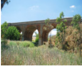
RAIL BRIDGE SOHE 2008
