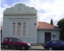
Coburg Court House
