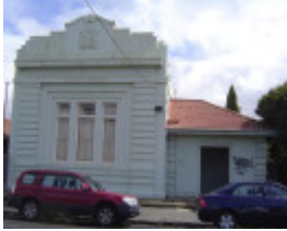
Coburg Court House
