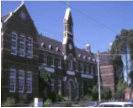
1 primary school number 1467 malvern road hawthorn front view nov1984
