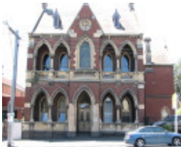
FORMER ES&A BANK (MANRESA PEOPLE'S CENTRE) SOHE 2008
