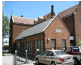
FORMER ES&A BANK (MANRESA PEOPLE'S CENTRE) SOHE 2008
