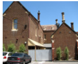
FORMER ES&A BANK (MANRESA PEOPLE'S CENTRE) SOHE 2008
