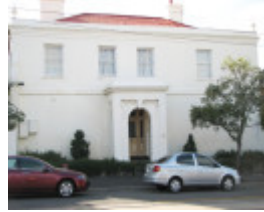
FORMER BRIDGE HOTEL SOHE 2008
