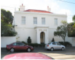
FORMER BRIDGE HOTEL SOHE 2008
