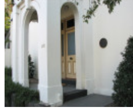
FORMER BRIDGE HOTEL SOHE 2008
