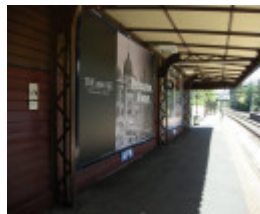
Looking south beneath the Platform 1 cantilever-truss canopy
