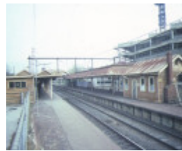
hawthorn railway station end view
