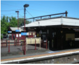
Looking from the west at the northern ends of the buildings and canopies on Platforms 1, 2 and 3
