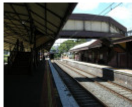
Looking northwards along the edge of Platform 2 with the south elevation of the roofed footbridge between the Platforms visible at upper right
