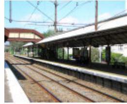
HAWTHORN RAILWAY STATION COMPLEX SOHE 2008
