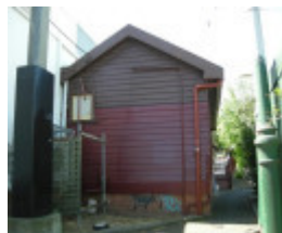
Platform 1 building - southwest elevation
