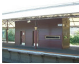
This building under the southern end of the Platform 2 and 3 canopy was constructed in 2014 and contains facilities for Protective Services Officers
