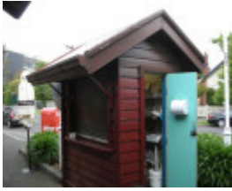
Small standalone building between Platform 1 building and Evansdale Rd
