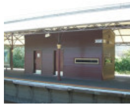
This building under the southern end of the Platform 2 and 3 canopy was constructed in 2014 and contains facilities for Protective Services Officers
