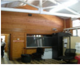
Looking south-west within the Burwood Rd end of the Platform 1 building
