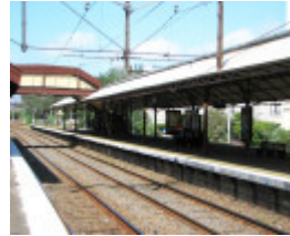
HAWTHORN RAILWAY STATION COMPLEX SOHE 2008
