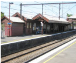
HAWTHORN RAILWAY STATION COMPLEX SOHE 2008
