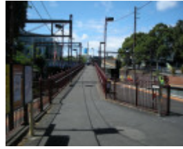
Looking north and upwards along the pedestrian walkway which links the island Platforms 2 and 3 with the south-side footpath on Burwood Rd bridge
