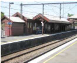
HAWTHORN RAILWAY STATION COMPLEX SOHE 2008
