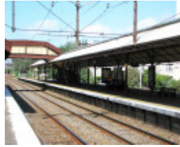
HAWTHORN RAILWAY STATION COMPLEX SOHE 2008
