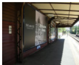
Looking south beneath the Platform 1 cantilever-truss canopy
