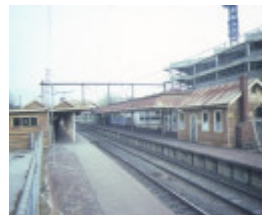
hawthorn railway station end view
