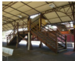
Access stairs to footbridge viewed from the southwest - from beneath the Platform 2 and 3 canopy
