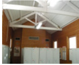
Looking north-east within the Burwood Rd end of the Platform 1 building - the king-post roof trusses about those of the platform canopy outside the wall to the left
