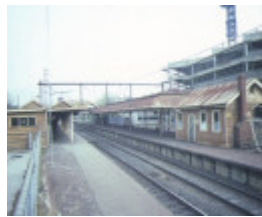
hawthorn railway station end view
