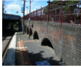
Looking north along Platform 3 at the west-facing brick wall beneath the walkway
