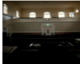
H01997 stawell courthouse gallery sep01 ac2
