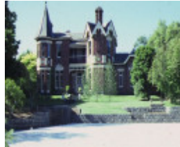
1 rotha 29 harcourt street hawthorn front view sep1981
