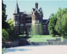
1 rotha 29 harcourt street hawthorn front view sep1981
