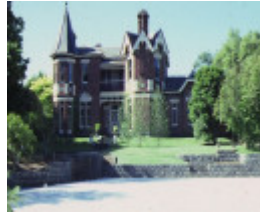
1 rotha 29 harcourt street hawthorn front view sep1981
