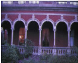
oxford isabella grove hawthorn arches along verandah
