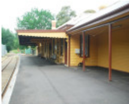
HEALESVILLE RAILWAY STATION COMPLEX SOHE 2008
