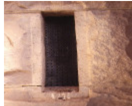
heathcote powder magazine slit window detail
