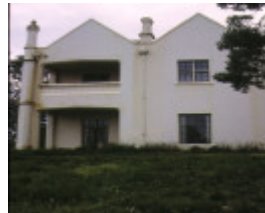
banyule heidelberg 1908 additions sep1995
