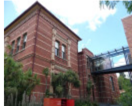
FORMER BALLARAT EAST FREE LIBRARY SOHE 2008
