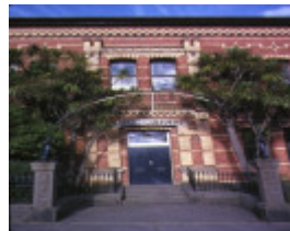
former ballarat east free library entrance detail jul1982
