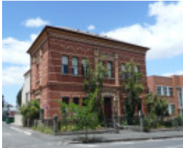
FORMER BALLARAT EAST FREE LIBRARY SOHE 2008
