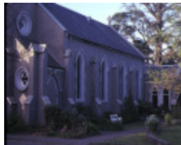
st johns anglican church heidelberg side view
