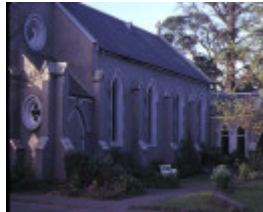
st johns anglican church heidelberg side view
