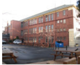
University High_parkville_rear elevation_Kj_9/7/08
