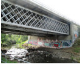
Bell Street Bridge
