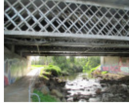
Bell Street Bridge
