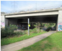
Bell Street Bridge
