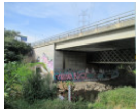
Bell Street Bridge
