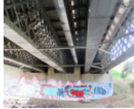
Bell Street Bridge
