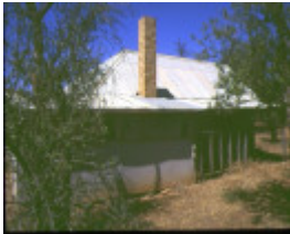
1 lake corrong homestead evelyn street hopetoun homestead rear
