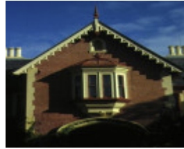
longerenong homestead jung via horsham detail front window
