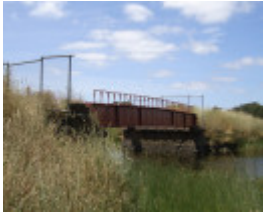
HOTSPUR BRIDGE SOHE 2008
