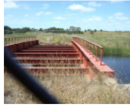
HOTSPUR BRIDGE SOHE 2008
