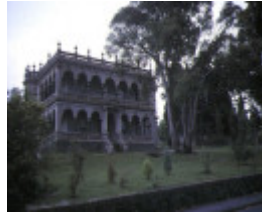
1 ravenswood ivanhoe front view
