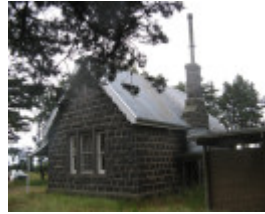
Former Leigh Shire Hall rear view
