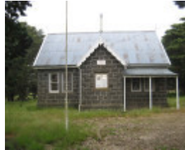
Former Leigh Shire Hall
