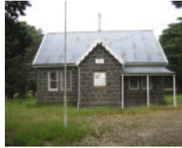
Former Leigh Shire Hall
