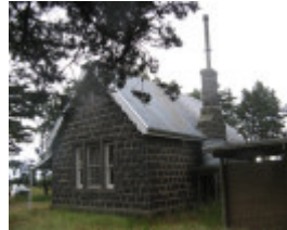
Former Leigh Shire Hall rear view
