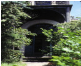
residence 12 jolimont terrace jolimont detail front entrance nov1980
