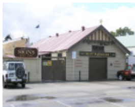
BLUNTS BOATYARD AND SLIPWAY SOHE 2008
