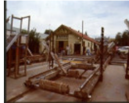
1 blunts boatyard slipway traverser & shed
