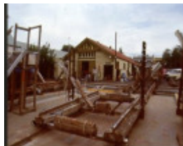
1 blunts boatyard slipway traverser & shed
