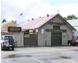
BLUNTS BOATYARD AND SLIPWAY SOHE 2008
