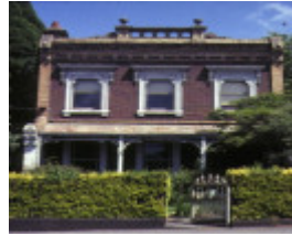
1 residence jolimont terrace jolimont front elevation nov1980
