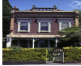
1 residence jolimont terrace jolimont front elevation nov1980
