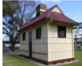
former grand rank cabman's shelter near footbridge yarra park jolimont side she project 2004
