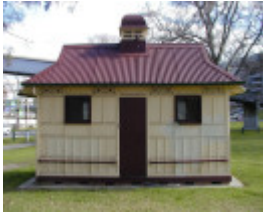
h00849 1 former grand rank cabman's shelter near footbridge yarra park jolimont front she project 2004
