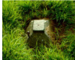
1 south base stone coverstone intact june01
