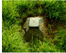
1 south base stone coverstone intact june01
