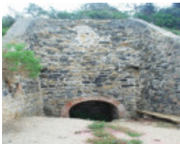
WALKERVILLE LIME KILNS SOHE 2008
