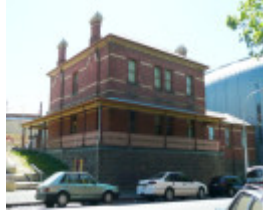
FORMER POLICE STATION SOHE 2008
