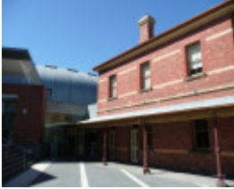
FORMER POLICE STATION SOHE 2008
