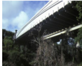
iron bridge maribyrnong river side elevation sep1984
