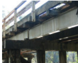
h00092 ol goulburn riv bridge seymour july 05 steel joists
