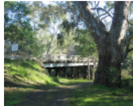
h00092 ol goulburn riv bridge seymour july 05 setting
