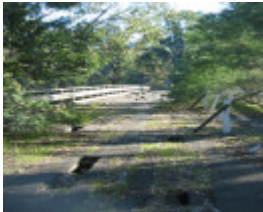
h00092 ol goulburn riv bridge seymour july 05 deck
