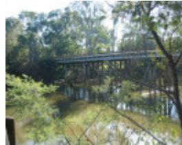
h00092 ol goulburn riv bridge seymour july 05
