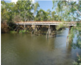
OLD GOULBURN RIVER BRIDGE SOHE 2008
