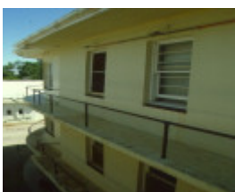
Former Mildura Base Hospital West Wing 2001
