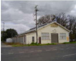
6168 Warragul Drill hall may07 ac 4
