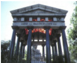
springthorpe memorial kew front view
