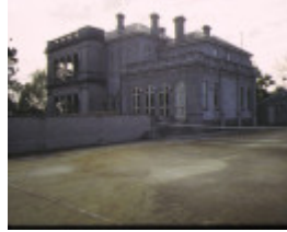
ross house kew rear view
