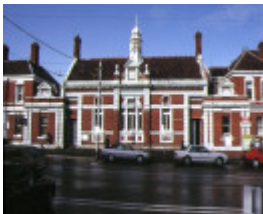
1 police station & former court house kew front view
