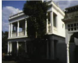
1 studley house kew front view
