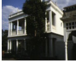
1 studley house kew front view
