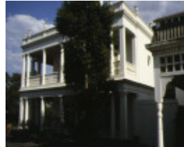
1 studley house kew front view
