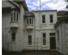
studley house kew rear view
