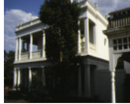
1 studley house kew front view
