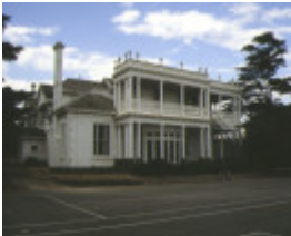
studley house kew side view
