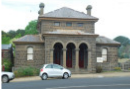
KILMORE COURT HOUSE SOHE 2008
