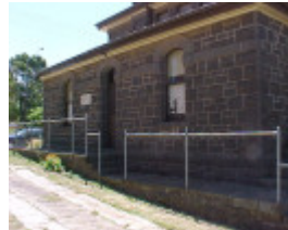
H01471 kilmore court house exterior side april 2003
