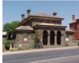
H01471 1 kilmore court house exterior april 2003
