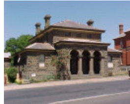
H01471 1 kilmore court house exterior april 2003
