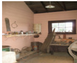
Interior - outbuilding west wing. Aug 2007.
