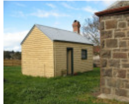
View of outbuilding. Aug 2007.
