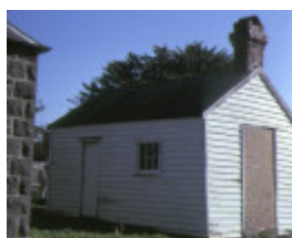
1 whitburgh cottage piper street kilmore outbuilding
