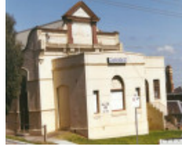
Photograph of the facade of the Rechabite Hall from High Street. The image shows the original Victorian parapet details as well as the later extensions to the front and side of the property. Source: Bunjil Place Connected Libraries. 1994. Rechabite Hall,
