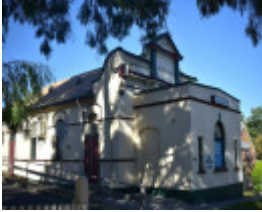
Oblique view of the Rechabite Hall facade and north eastern side.
